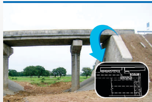
True Geogrid reinforced soil bridge abutment
