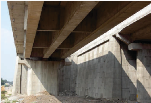
15.5m high single tier geogrid reinforced soil wall with discrete panel facing.
