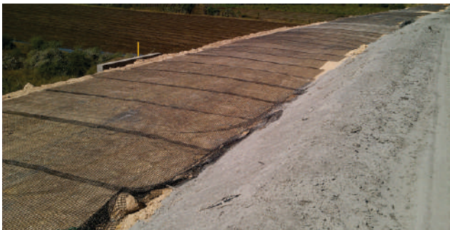
Stage 1: Geogrid reinforcement laying in progress
