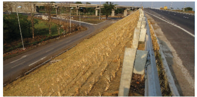
Stage 2: Vetiver grass sowing in process
